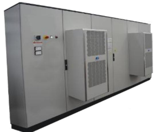
The switch cabinet is equipped with thermal conditioning system.
